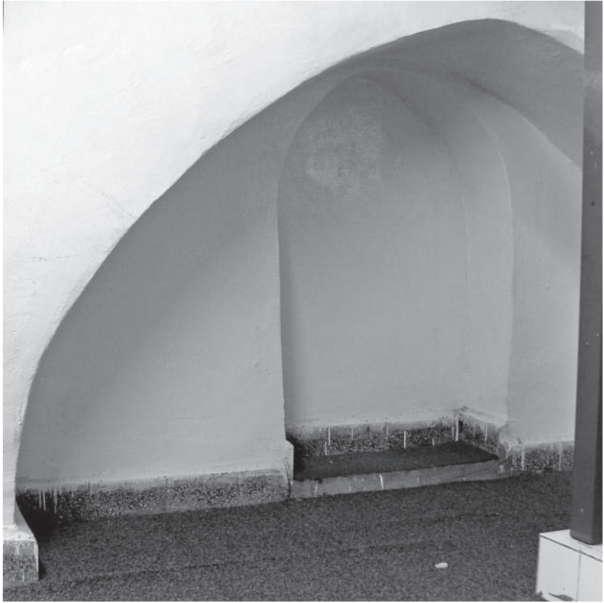
Figure 3.48 Blind arches in north wall of crypt of mausoleum of Asma', Maymuna and Hamida. Photo: Author
