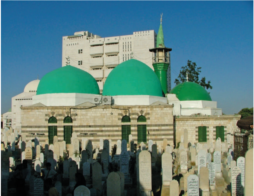
Figure 3.9 Western elevation of mausoleum of Sukayna and Umm Kulthum and mausoleum of the Qalandariyya. Photo: Author
