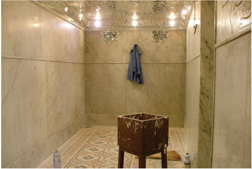
Figure 3.11 Hallway in crypt of Sukayna and Umm Kulthum, view from stairway, facing east. Doorway to crypt of Umm Kulthum is visible on right. Renovation was underway when these photos were taken. Photo: Author
