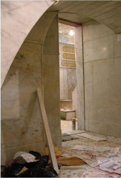
Figure 3.14 View of multiple phases of buttressing, looking out door towards hallway from inside crypt of Sukayna. Renovations often appear to be ongoing. Photo: Author
