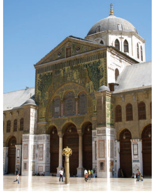
Figure 4.6 Transept of the prayer hall, Umayyad mosque. Photo: Author
