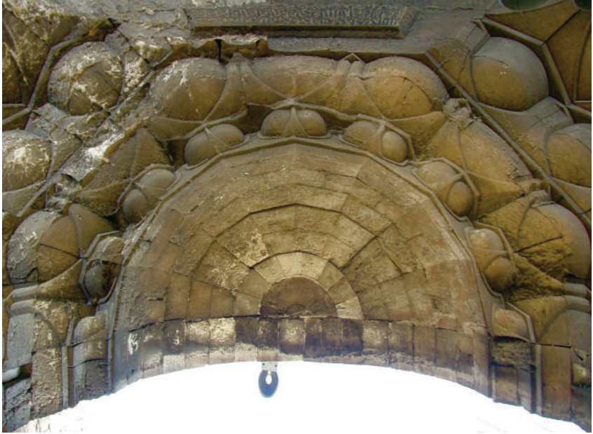
Figure 2.6 View upward into stone muqarnas dome over entrance. Photo: Author
