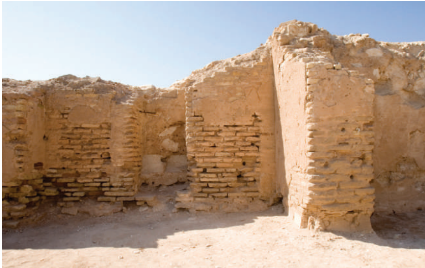
Figure 1.20 Mihrāb niche cut into south wall of prayer hall, south-east corner. Photo: Drew Stauss, Departure Studio
