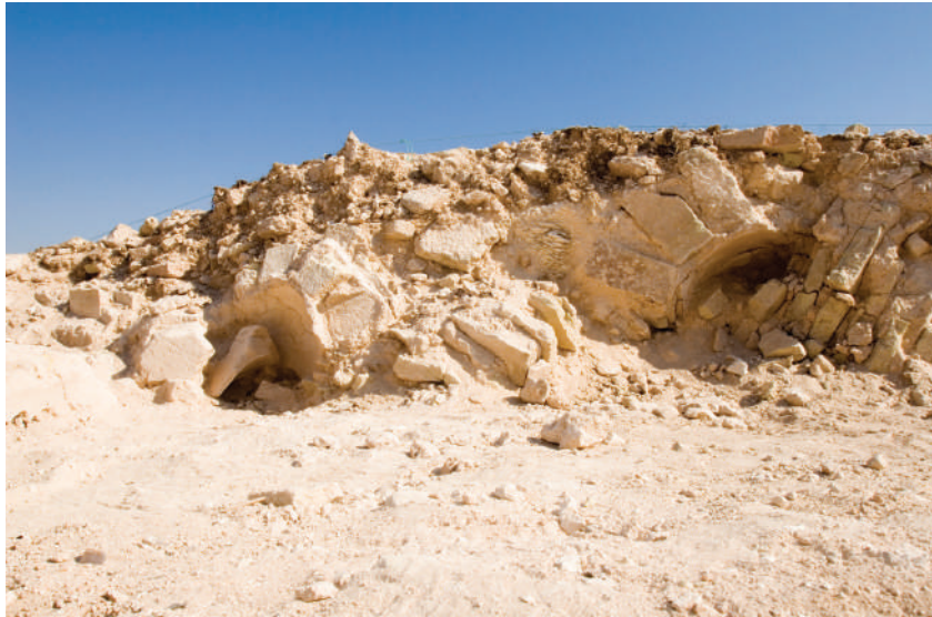
Figure 1.33 Fallen squinches in rubble of doorway. Photo: Drew Stauss, Departure Studio
