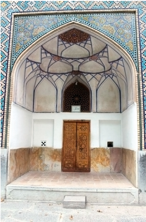
FIGURE 19 The Madrasa-yi Sulṭānī. Exterior view of typical chamber porch.
