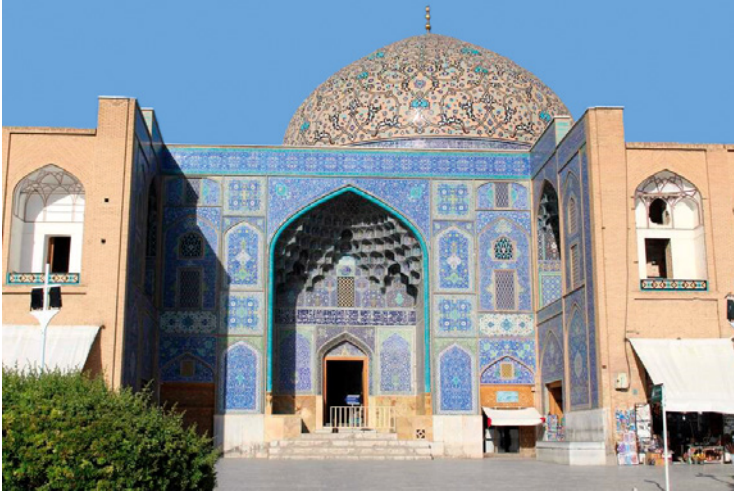
FIGURE 10 View of portal and dome from west. Masjid-i Shaykh Lutfullāh.
